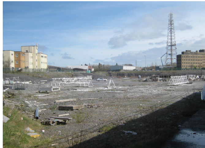
Existing Site View North
