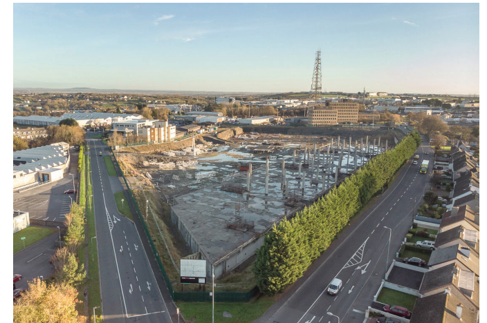
Existing Aerial View North
