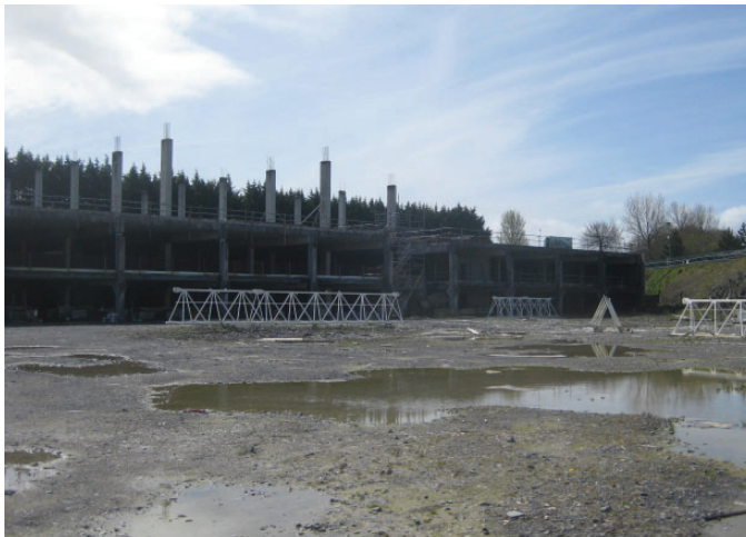
Existing Site View South
